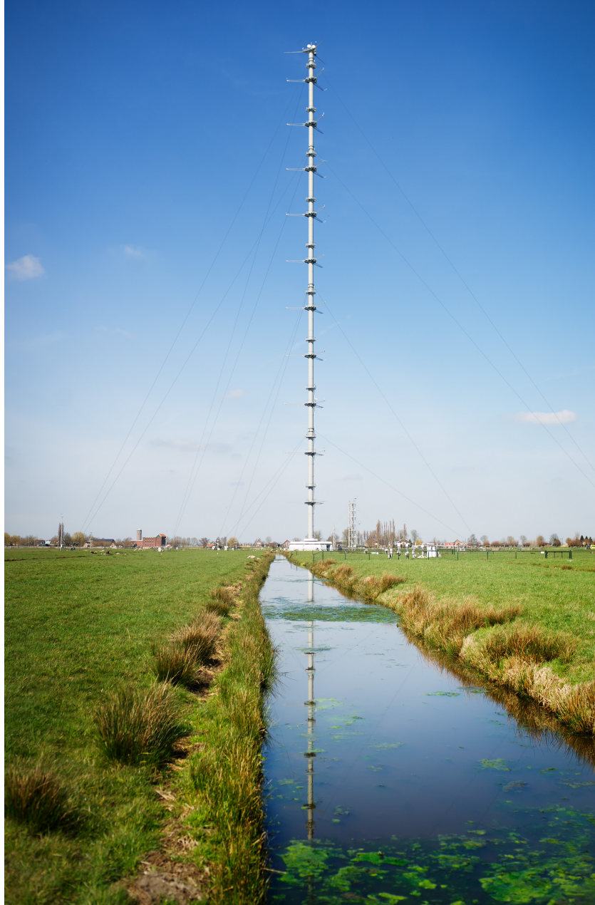
Figure 2: The 213-m tall Cabauw meteorological mast (photo by Ruben Jorksveld, KNMI).
